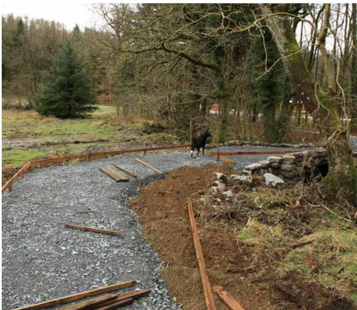
The level of the finished path surface had to be carefully marked out with wooden boards.
