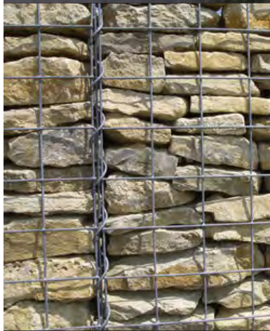
STONE GABION WALLS
