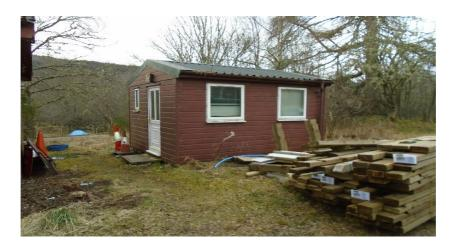
**Building 3** - workshop, size = 12.3m x 5m, consists of large workshop area & separate store room. Not in use, deemed unsafe. Evidence of leaking roof, false ceiling fitted, possibly creating condensation, caused by poor ventilation. Electric supply disconnected, evidence of a wood burning stove(only the chimney remains.)
