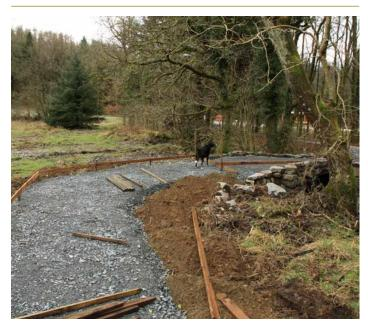
The level of the finished path surface had to be carefully marked out with wooden boards.
