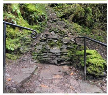
Small landslips are stabilised with walls built from local stone, so they blend in with their surroundings.
