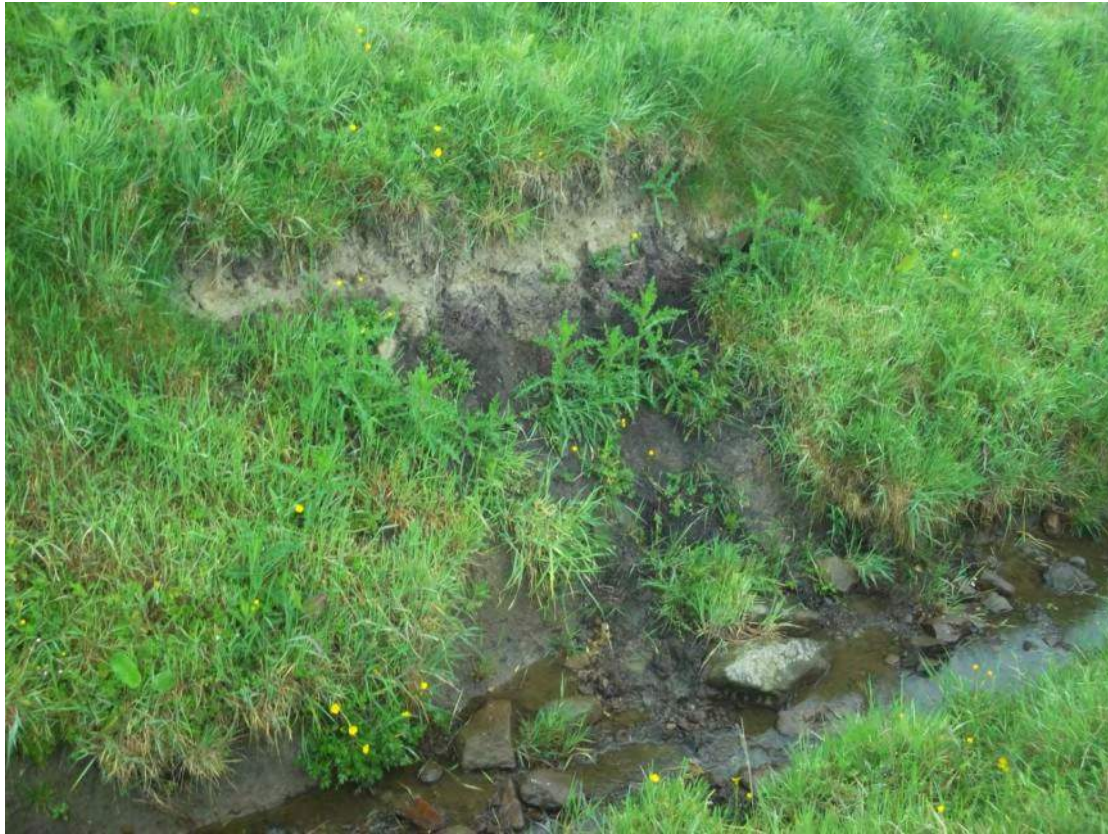
Figure 11 – Bank of field drain along field 17 showing underlying drift geology.
