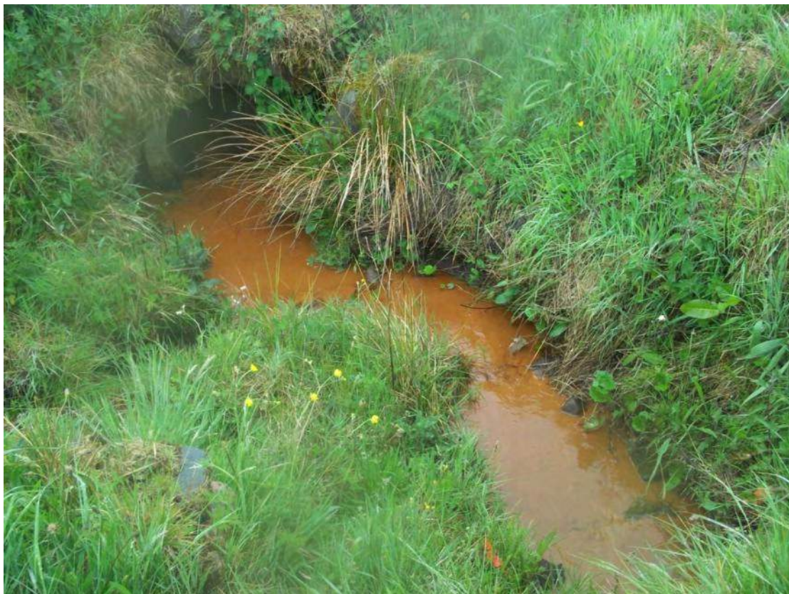
Figure 18 – Field drain at southern end of field 23 showing water discolouration.
