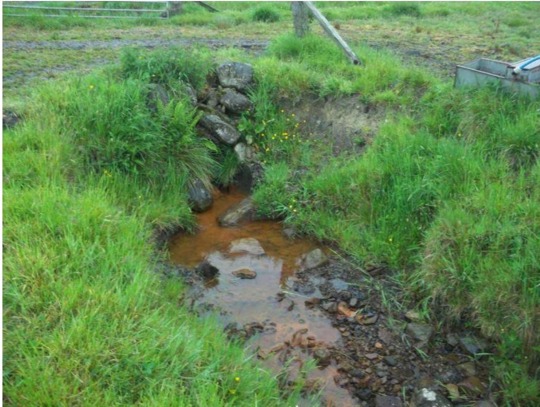
Figure 9 – Field drain exiting culvert under track at boundary of fields 17 and 24.
