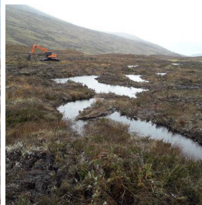
Figure 5b. Re-profiling of peat hags and the resulting higher water table.
