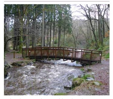
A bridge on the trail had to be designed to allow plenty of space for the burn in spate, but without too steep a gradient.
