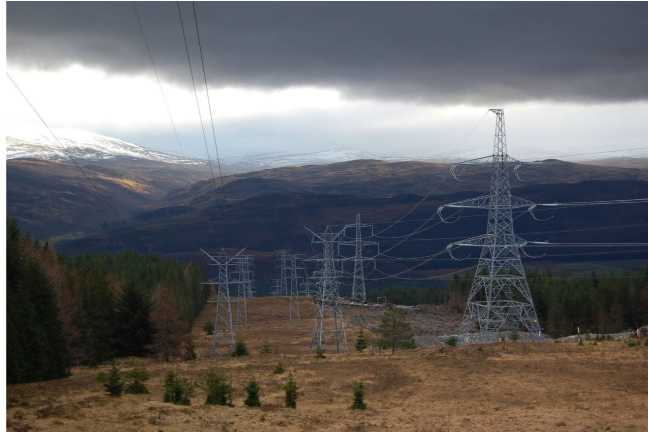
The Beauly-Denny powerline and wayleave corridor with (currently) strong linear forest edges
